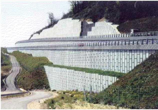
Fig. 1: The Tèche retaining wall
